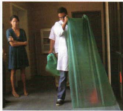
The film containing the encapsulated contamination can then be peeled off and disposed of.
